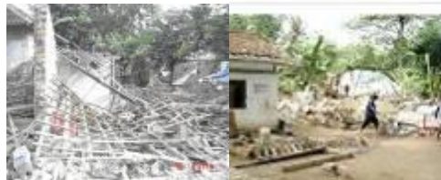
Fig. 3 & 4. Destruction under Earthquake in Bantul, Yogyakarta (May-2006)
