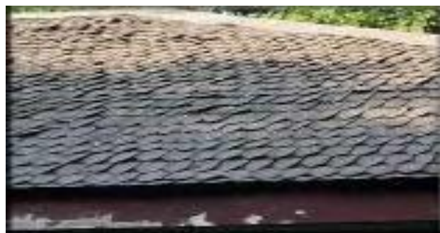
Fig. 9. 35 year old roof in Surabaya.
