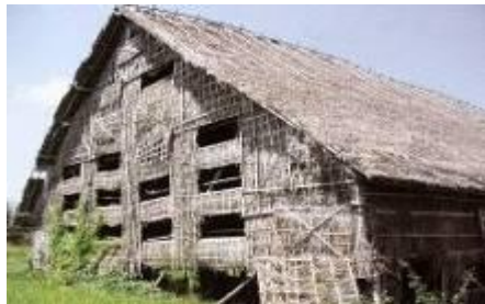
Fig. 8. Traditional warehouse in Bantul which is highly resistant to the earthquakes.
