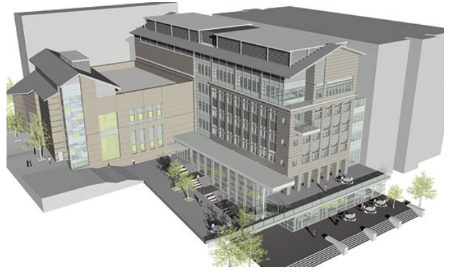
Fig. 4. Sutardja Dai Hall is 141,000-square-foot building, and our BRITE-S testbed is within this building.
