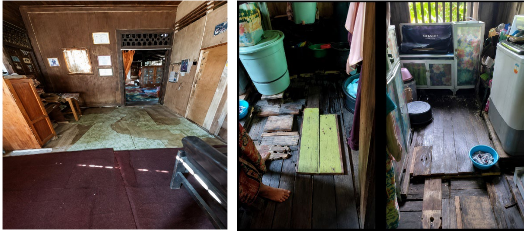
Fig. 5. Plank Floor Covered with Plastic Mat/Carpet and Patchwork Repairs (Author, 2023).
