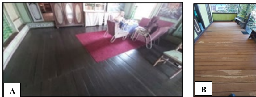
Fig. 4. The Ironwood Floor, which Remains Clean and Shiny (A); Newly Replaced Ironwood Floor (B) (Author, 2023)
