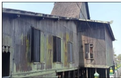
Fig. 2. The Exterior Walls of the House Made of Ironwood Board, which Remains in Good Condition (Author, 2023)
