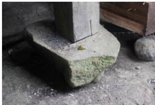
Figure 2. Stone used as the foundation [9]
