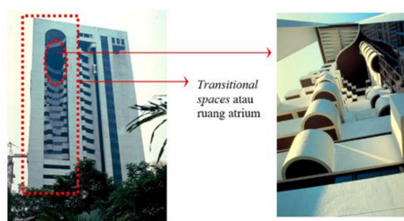
Fig 8. Atrium in modern buildings as the adoption of vernacular architectural features in anticipating the local climate in increasing comfort.
