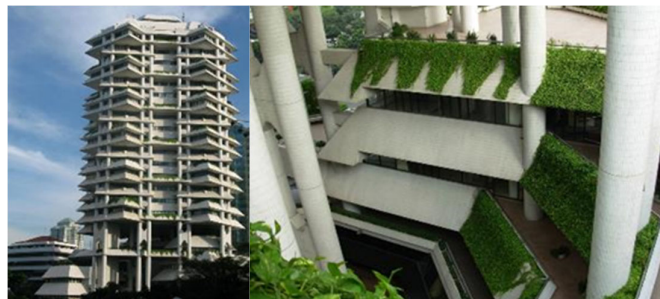
Fig 4. Wisma Dermala: A large balcony and elements of vegetation to create air circulation and create a microclimate
