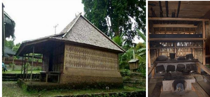
Fig 6. The high floor of the building and the walls of woven bamboo in anticipation of the heat of the soil and create airflow and sunlight. This reduces the use of excessive energy during the day.
