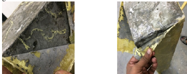
Figure 12: Failure Patterns of RC Short Columns Strengthened by AFRP sheets
