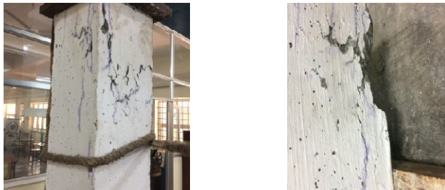
Figure 9: Failure Patterns of Reference RC Short Columns
