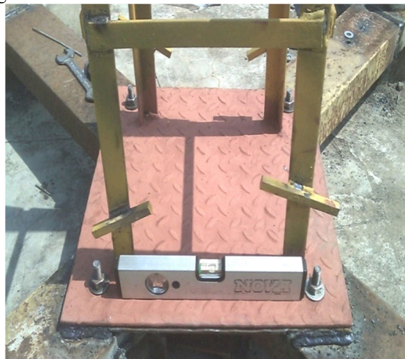
Fig. 12. Erection of Tower
