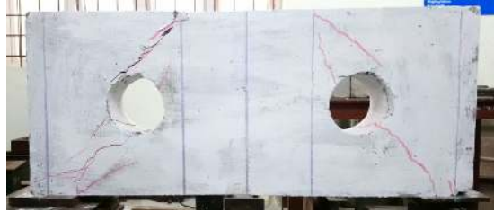
Figure 10 Crack Pattern Observed in Deep Beam with Circular Opening
