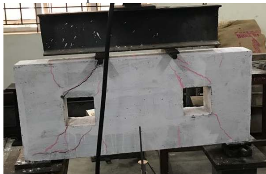
Figure 8 Crack Pattern Observed in Deep Beam with Square Openings
