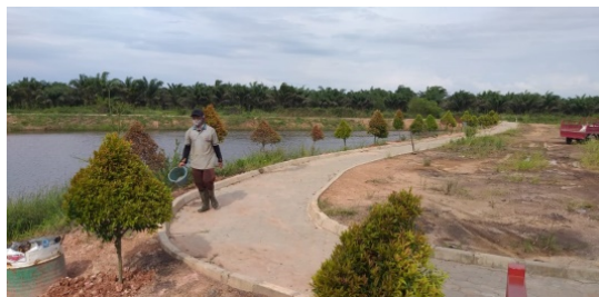
Figure 7. Paving block road.
