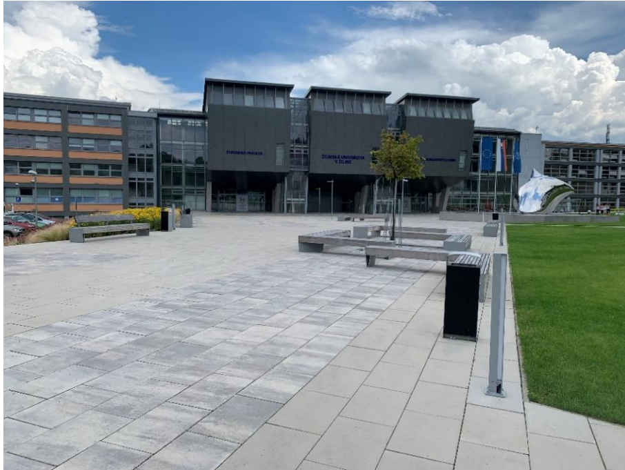
Fig. 2. A front view of the campus and the Rectorate's building
