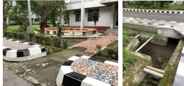
Fig. 7. Pedestrian safety level is seen from the condition of the level height and the proximity of the open drain.
