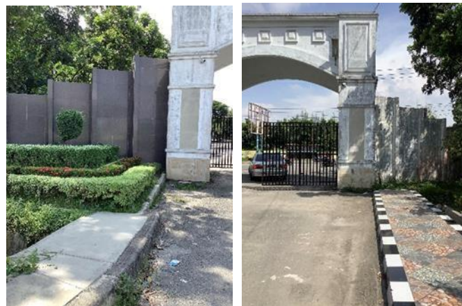
Fig. 5. Pedestrians access is cut off between campus and public pedestrian platform.
