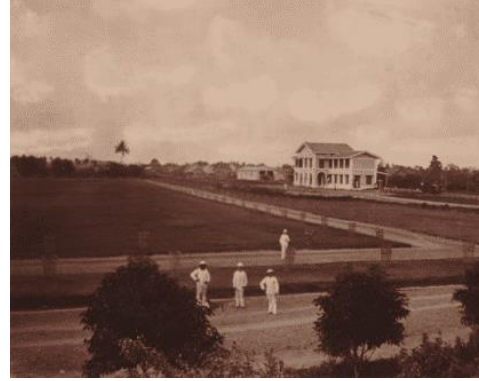
Fig. 2. Esplanade During Early Construction in 1886 [10].
