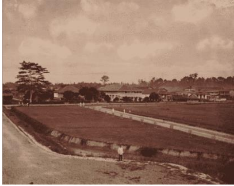
Fig. 1. Esplanade During Early Construction in 1886 [9].
