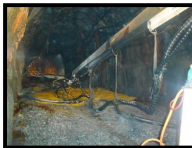
Fig. 5. Taking of Rebound Data on Shotcrete
