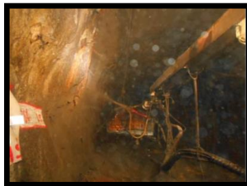
Fig. 3. Spraying Shotcrete at GC2760 Track 20
