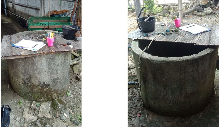
Figure 3. One of the features of a dug well (W8).
