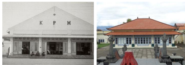
Fig. 6. SMPN I Singaraja Building
