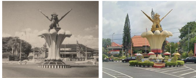
Fig.3. Buleleng Regent Office
