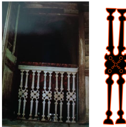
Figure. 11: Window lattice wood carving of Rumah Bumbung Panjang in Perlis. (Resource: Abdul Halim Nasir, 2016 [41]; Illustration: Researcher)
