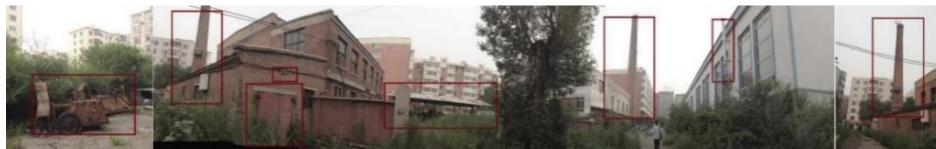
Fig. 1. Former site of Harbin Welding Research Institute.
