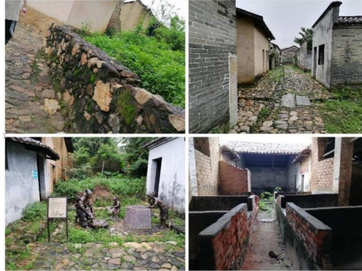
Figure 1 Current situation of traditional village architecture and landscape in Conghua
