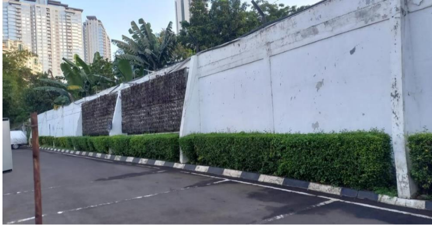
Fig. 2 Location of Biogas Lamp: Drop Off at Universitas Pertamina
