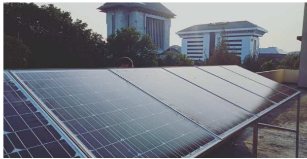
Fig. 1. Solar Panel Installation.
