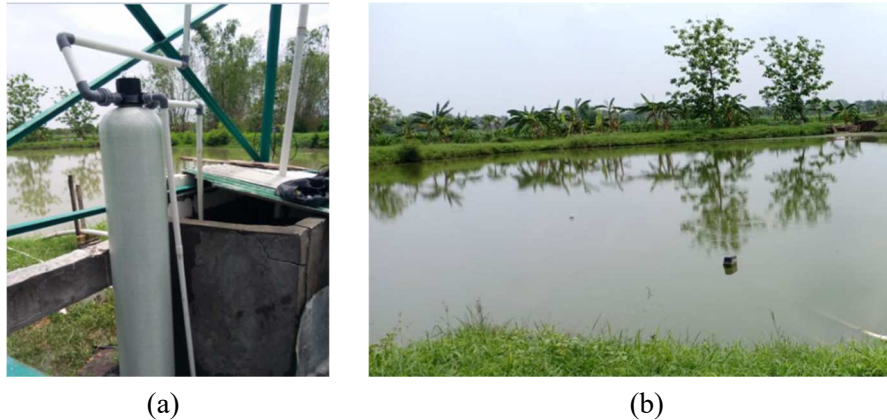
Fig. 3. (a) Water treatment equipment, (b) Karangasem Lake (Sirnobojo village)
