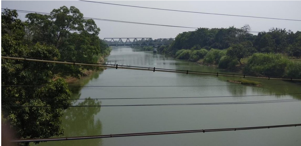
Fig. 2. The Cimanuk river conditions in West Java
