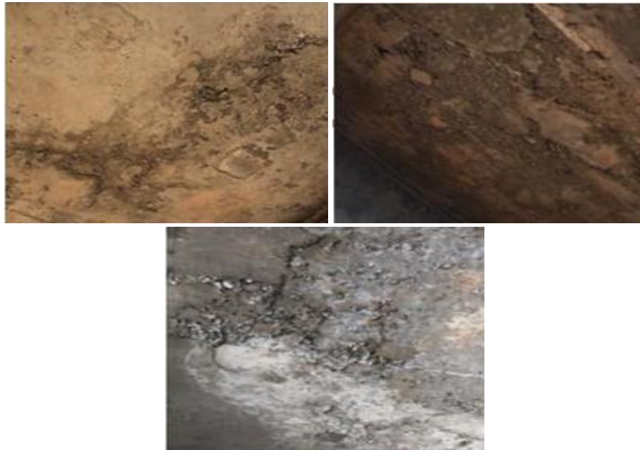
Fig. 1. Slab trestle elemental visual condition
