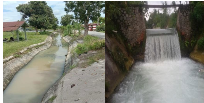
(a). Sewer flow channel (b). Dam pouring channel Figure 1. Types of limited and fixed channels in picohydro applications
