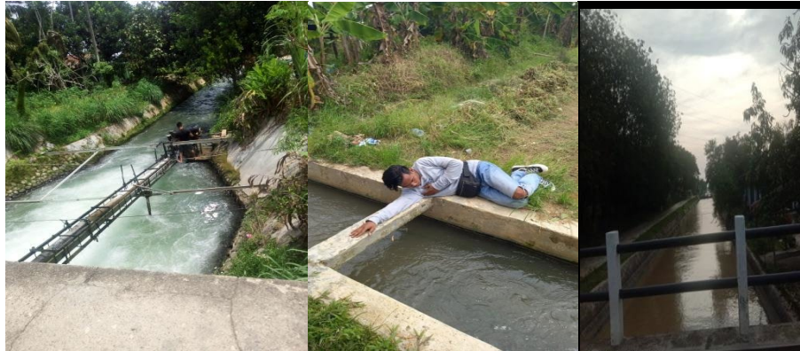
Figure 6. Measurement application and potential installation of pico-hydro irrigation flow
