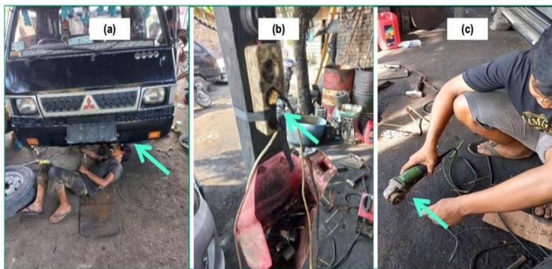
Figure 1. Potential hazards to the car repair work: (a) the work of raising the car to the car lift, (b) electrical conditions, and (c) using a grinding machine.
