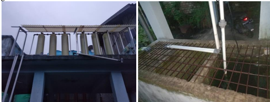
Fig. 6. Installing a filter tool from the government
