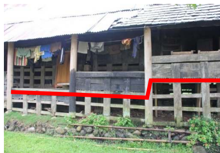
Fig. 7. Construction structure in Banua Layuk is in form of interlocking construction
