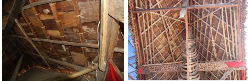
Fig. 4. Open Ceiling in Banua Layuk Roof Frame
