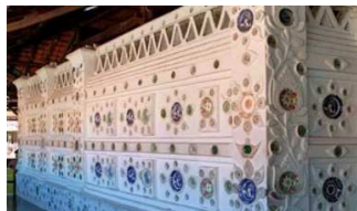
Figure 14. The wall surface of Sunan Gunung Jati Mausoleum
