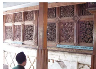
Figure 8. The wall surface of Sunan Drajat Mausoleum
