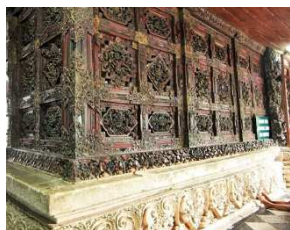
Figure 7. The wall surface of Sunan Giri Mausoleum in Sunan Giri Mosque site
