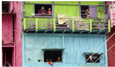
Figure 3. Bamboo as one of material building
