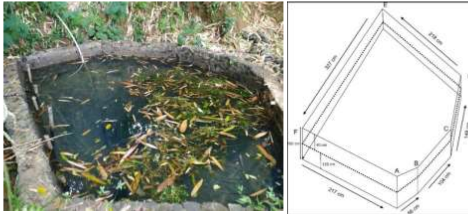
Fig. 3. the structural protection shape bordering the Ngureng spring outlet
