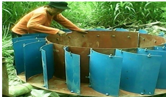
Fig. 2. The assembly process in the W2KDS test site
