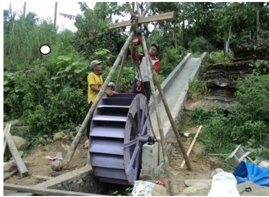
Fig. 7. Installation of the W2KDS on the ground
