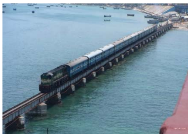
Figure 3. Railway Bridge demonstrating event: train passing over bridge
