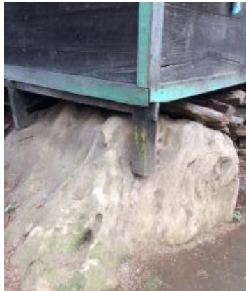
Fig. 2. The tie between foundation and column.
