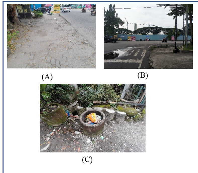
Fig. 3. Documentation of Facilities in the Teladan Stadium area.
