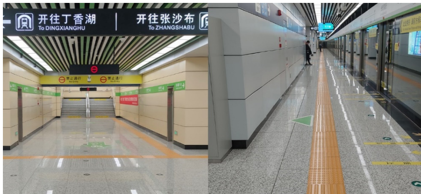
Fig. 2. Blind sidewalks which seem reasonable but have problems (Source of figure: taken at the scene by author)
