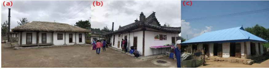
Fig. 4. — Houses. a. Thatched roof house. b. Tile roof house. c. Coloured steel roof house.
