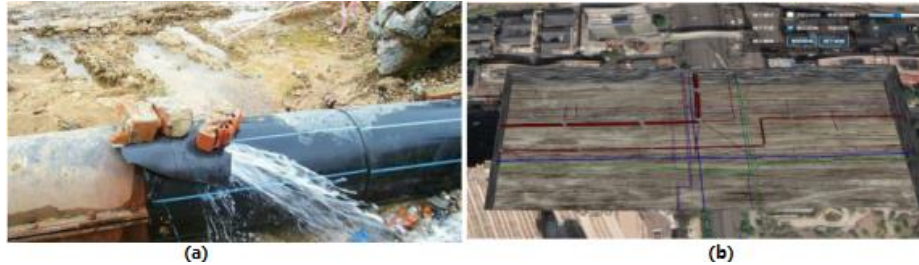
Fig. 1. (a) Water Pipe Break Photograph, (b) 3D GIS based on the water supply network in BS
