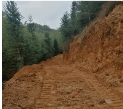
Figure 3. Temporary road in mountainous areas.
