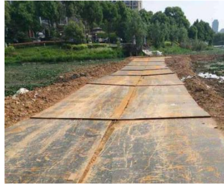
(b)Laying steel plates
