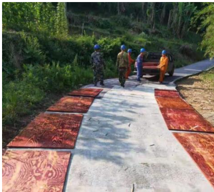
(a) Laying boards
