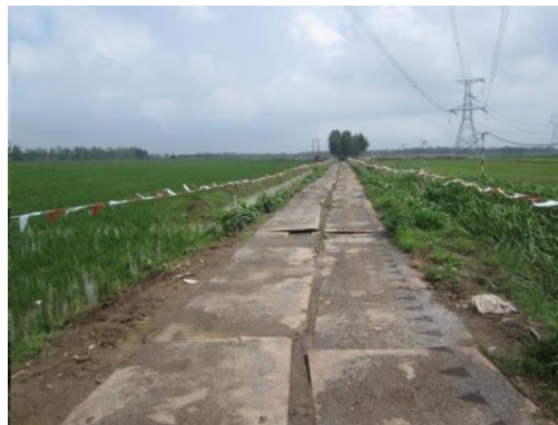
Figure 4. Temporary road boundary restriction
