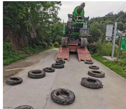
(b) Laying tires
