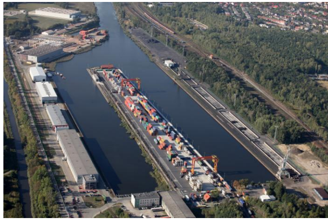
Fig. 7: Multimodal terminal Śląskie Centrum Logistyki SA, Gliwice, Poland [9]
