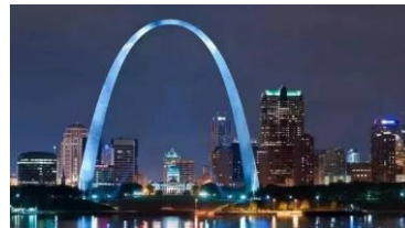
Fig. 5. Jefferson Memorial Arch
