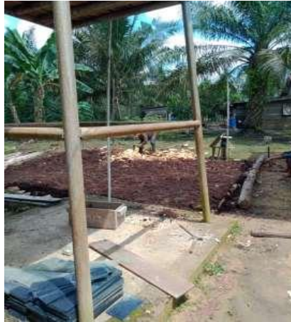
Figure 6. Construction of a peat water purification installation site in Dusun 1
