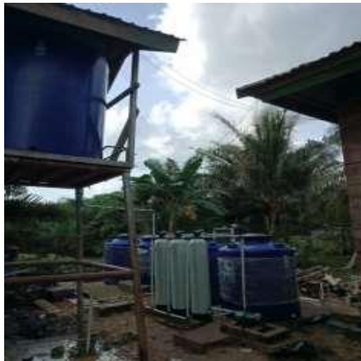
Figure 7. Assembly of peat water purification installation (Dusun 1)
