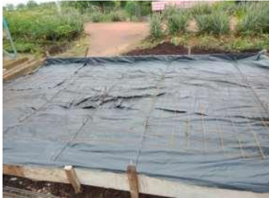
Figure 5. Construction of a peat water purification installation site in Dusun 3
