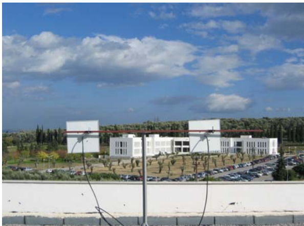
Figure 1. The 27dBi patch pannels at the roof of FORTH on the mounting pole used.
