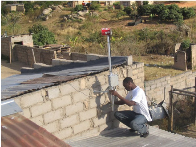
Fig. 4. Installation of a DIY kit for wireless communications, provided by the Meraka Institute of CSIR
