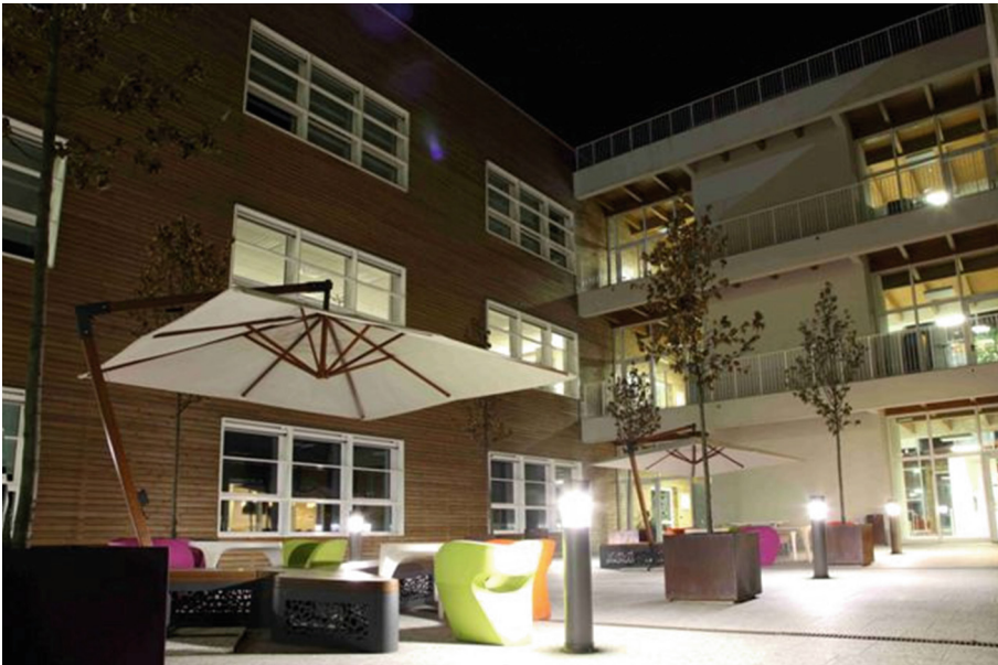
Fig. 5. The inside of Building 03 - Garretti Associati
