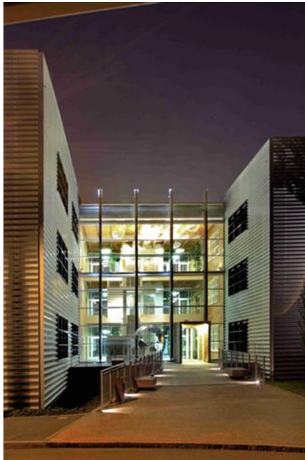
Fig. 4. The outside of Building 03 - Garretti Associati
