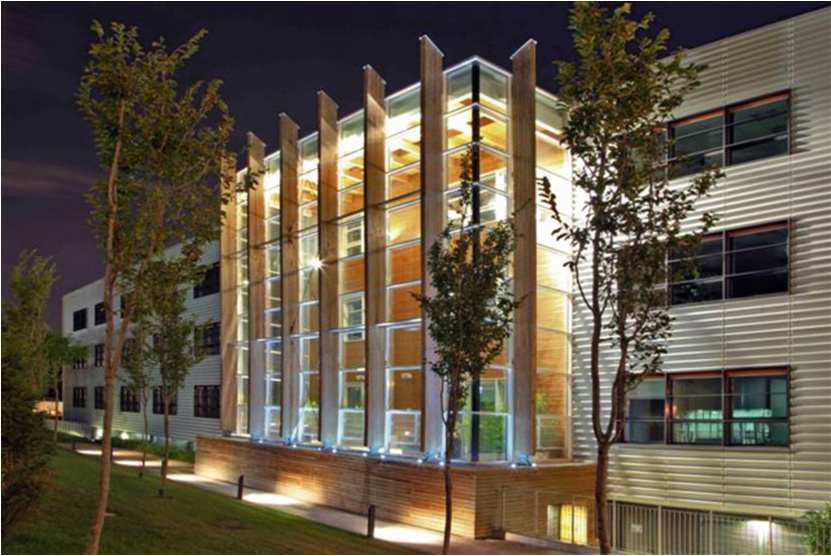
Fig. 3. The outside of Building 03 - Garretti Associati
