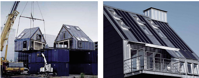
Fig. 2. SOLTAG project - prefabricated system [3]
