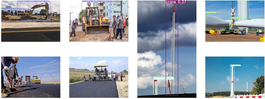
Fig. 4. Examples of detected objects by YOLOv3-SPP after re-training with our annotated images from wind turbine construction videos. Instances of the class “foundation building machines” (e.g. excavator) are as well detected on road construction images.
