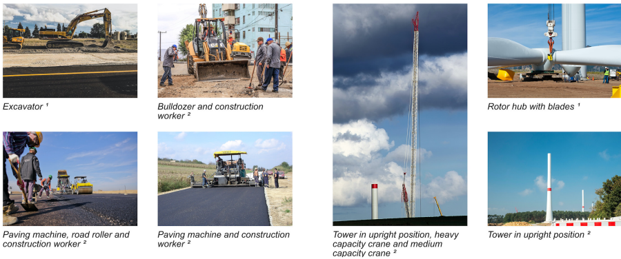
Fig. 1. Example scenarios: road construction (left) and wind turbine assembly (right). Most process steps involve a different set of vehicles, machines, materials or parts that can be observed on the image. A person familiar with the process often can identify the currently performed process step by observing only a single image. 1 sample images from unsplash.com , 2 sample images from pixabay.com
