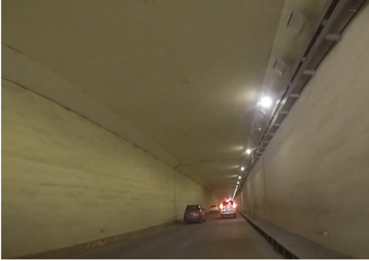
Fig. 2. Rectangular tunnel with two lanes
