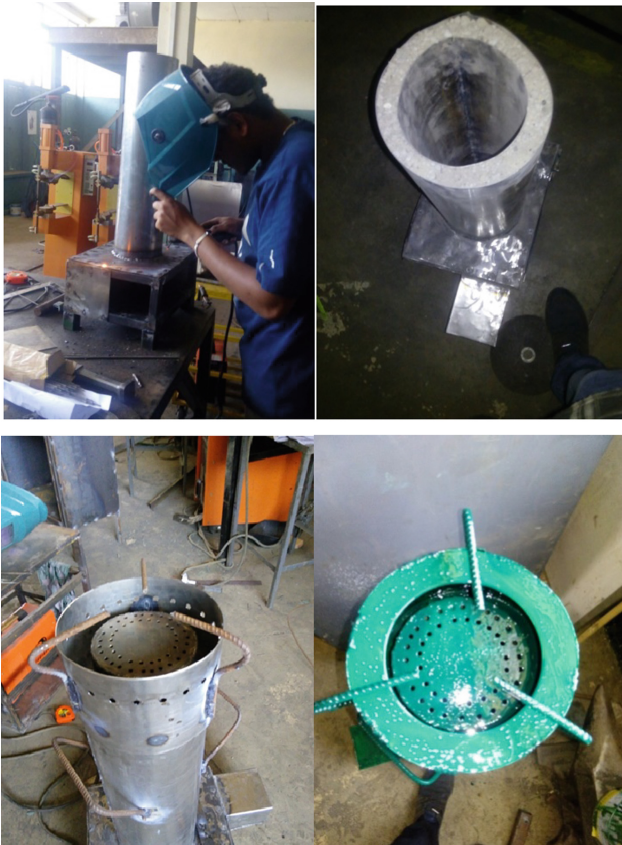
Fig. 3. Gasifier stove while construction.
